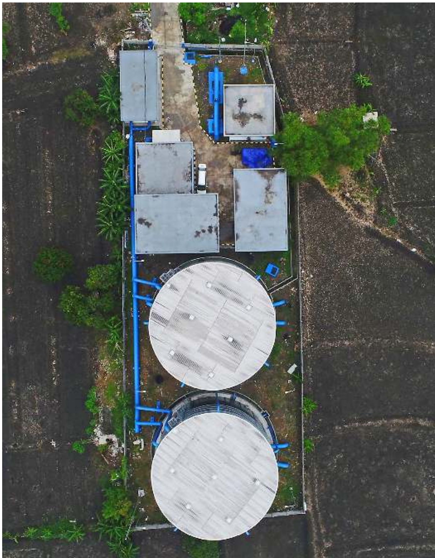
PIPA JARINGAN SPAM UMBULAN
